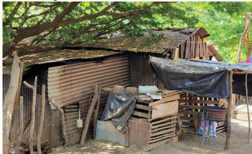
Before construction: many homes in El Platanal are built with corrugated tin and fragile materials, leaving families vulnerable during hurricanes and severe storms.
