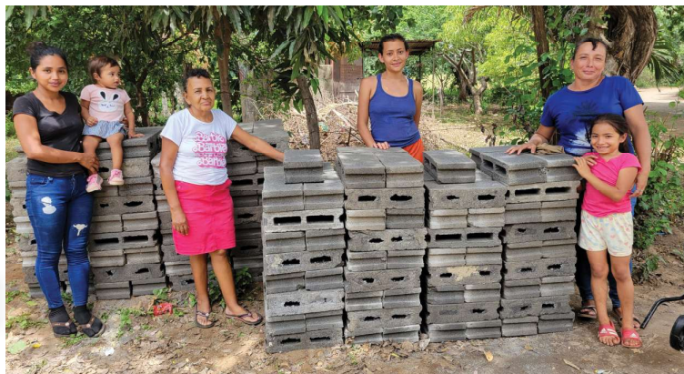
Above - Women from the community stand beside the cinderblock materials that will be used to build new latrines, part of an initiative focused on improving sanitation and dignity for local families.
